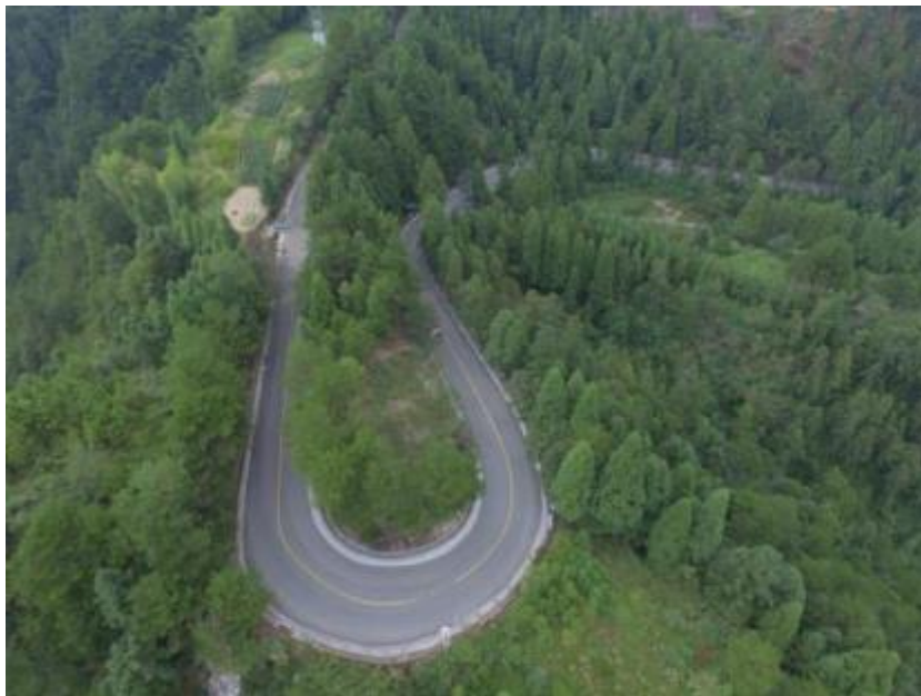
Figure 6.333 – The full view of the road before any measures
