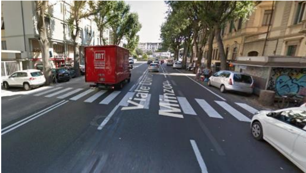
Figure 6.137 – Pedestrian crossing before the intervention [2]
