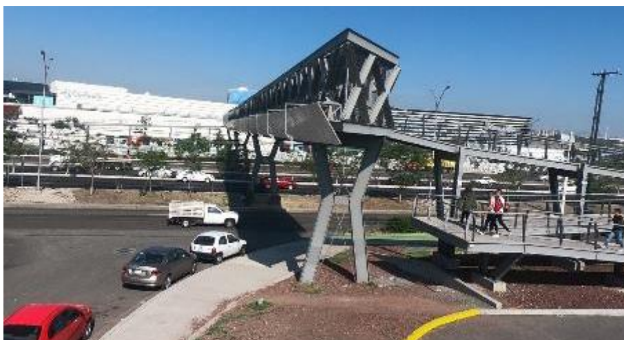
Figure 6.94 - Side view of the Pedestrian Crossing-Grade Separation, seen from the east side
