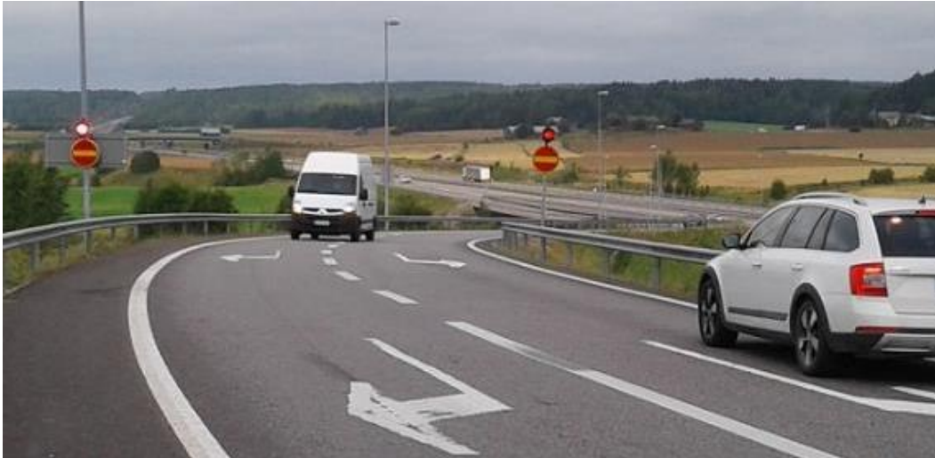
Figure 6.204 - The most significant system developed in the new project was a warning light that turns red if a driver is about to take a motorway ramp in the wrong direction. Photo: Jaakko Klang
