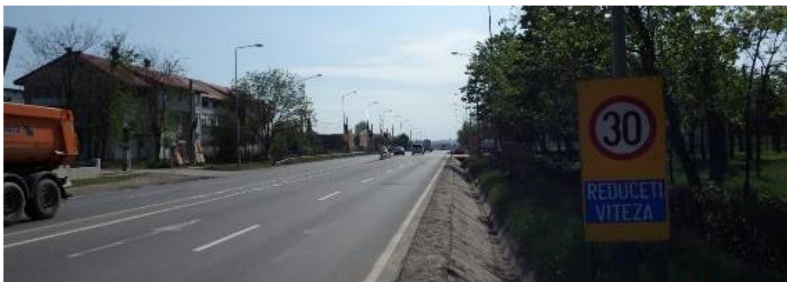
Figure 6.364 – After the intervention. Road view before the turning point
