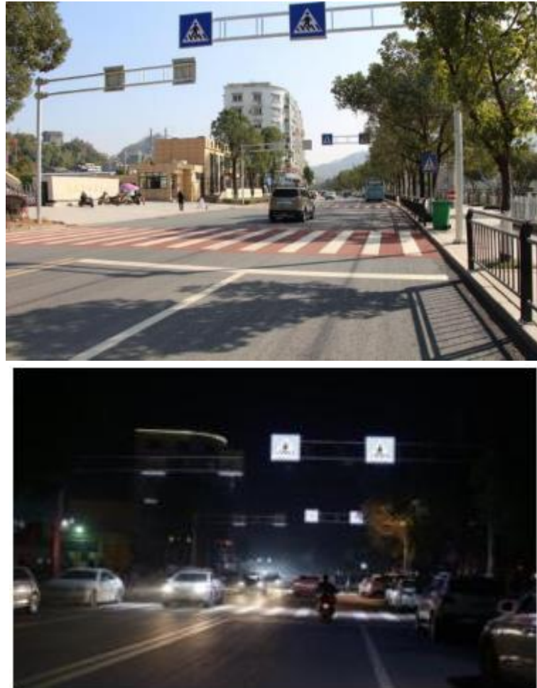
Figure 6.5 - Setting 2 sets of LED lighting facilities and active light-emitting traffic signs
