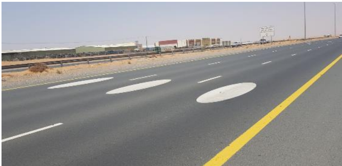
Figure 6.289 - White dots to keep safety distance. Sheikh Mohammed Bin Zayed Road (Umm Al Quwain). Detail 2
