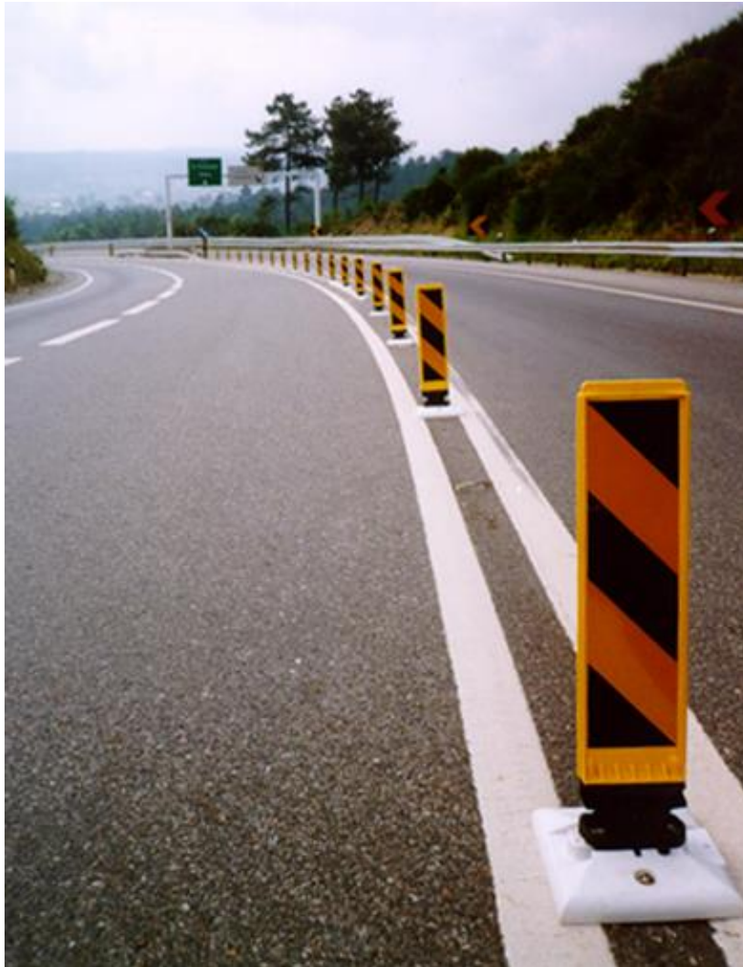
Figure 6.167 – Type O7 plastic position marker posts at the road axis
