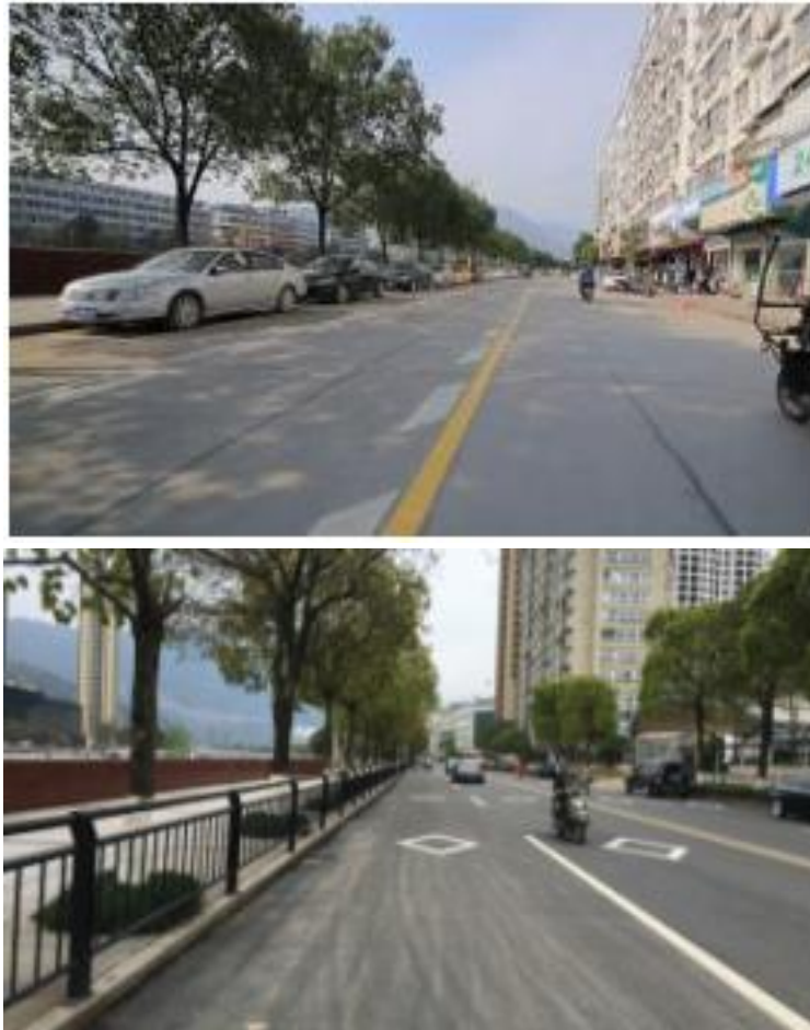
Figure 6.6 - Setting up the pedestrian barrier
