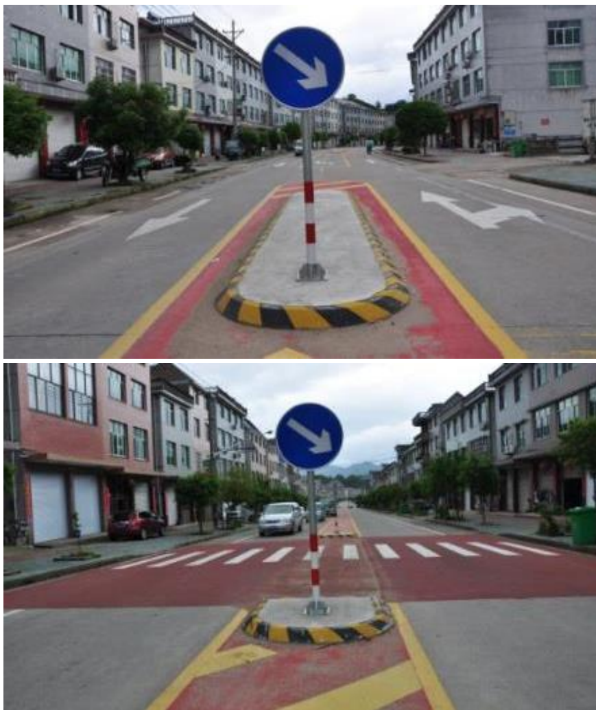
Figure 6.9 - Set up a pedestrian refuge island
