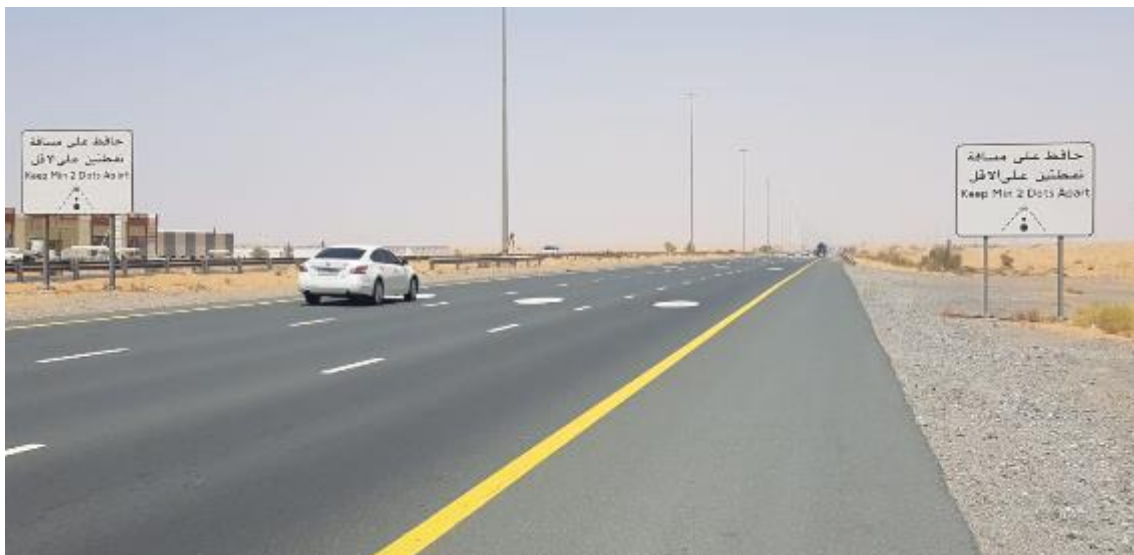
Figure 6.291 - White dots to keep safety distance. Sheikh Mohammed Bin Zayed Road (Umm Al Quwain). Detail 4
