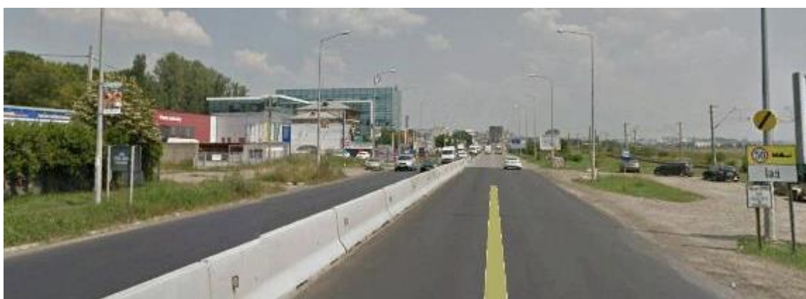
Figure 6.111 – During the intervention: construction site section 2, Iasi oriented view
