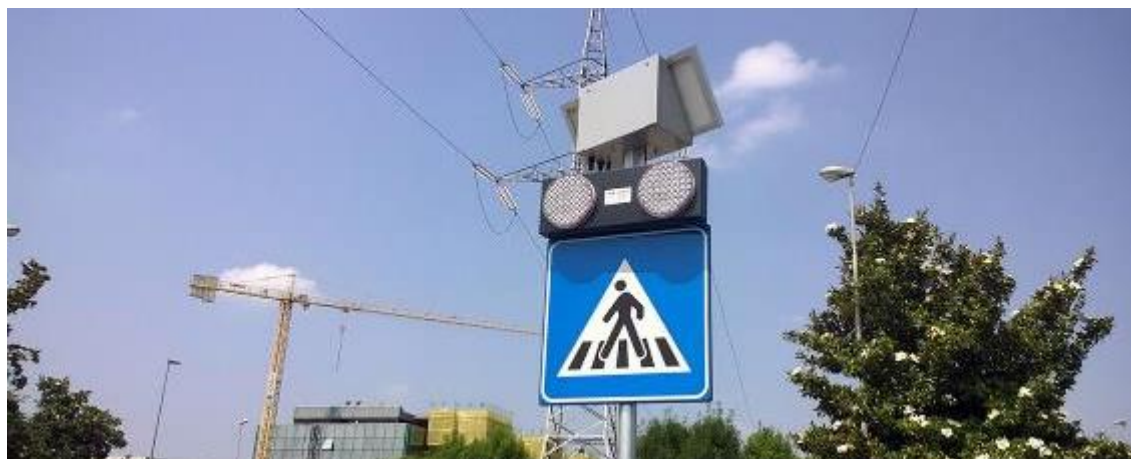
Figure 6.82 - Photos showing the cycling crossing, vertical road signs, and flashing traffic lights at the project junction following the first phase completion (May 2014)
