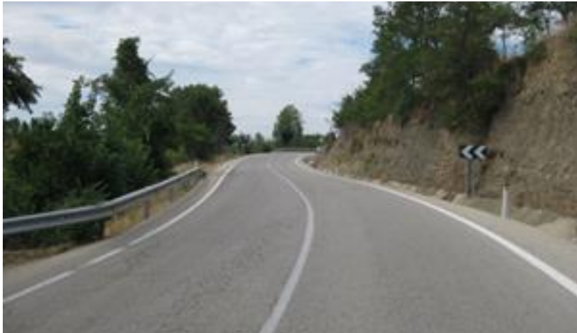
Figure 6.278 - Example. Junction without sight because cut slope
