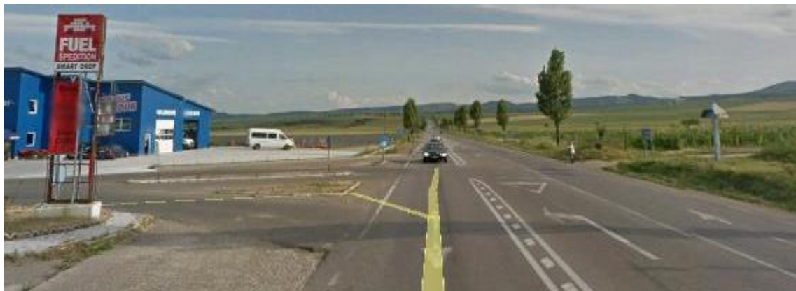
Figure 6.178 – View from the road after the intervention, closer to the intersection 1
