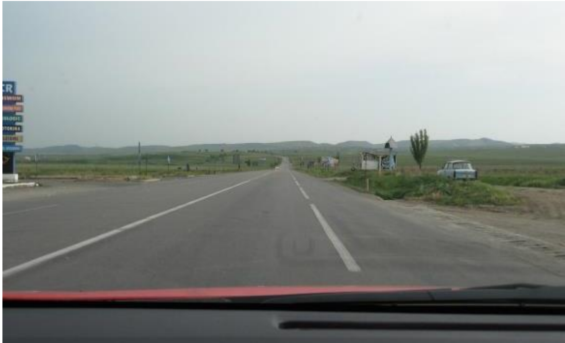
Figure 6.176 – View from the road before the intervention, closer to the intersection
