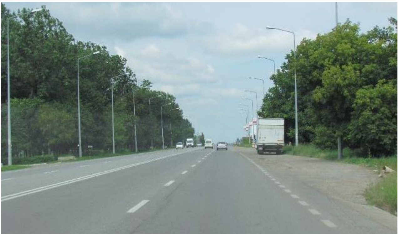
Figure 6.359 – Before the intervention. Road view before the turning point, section 2
