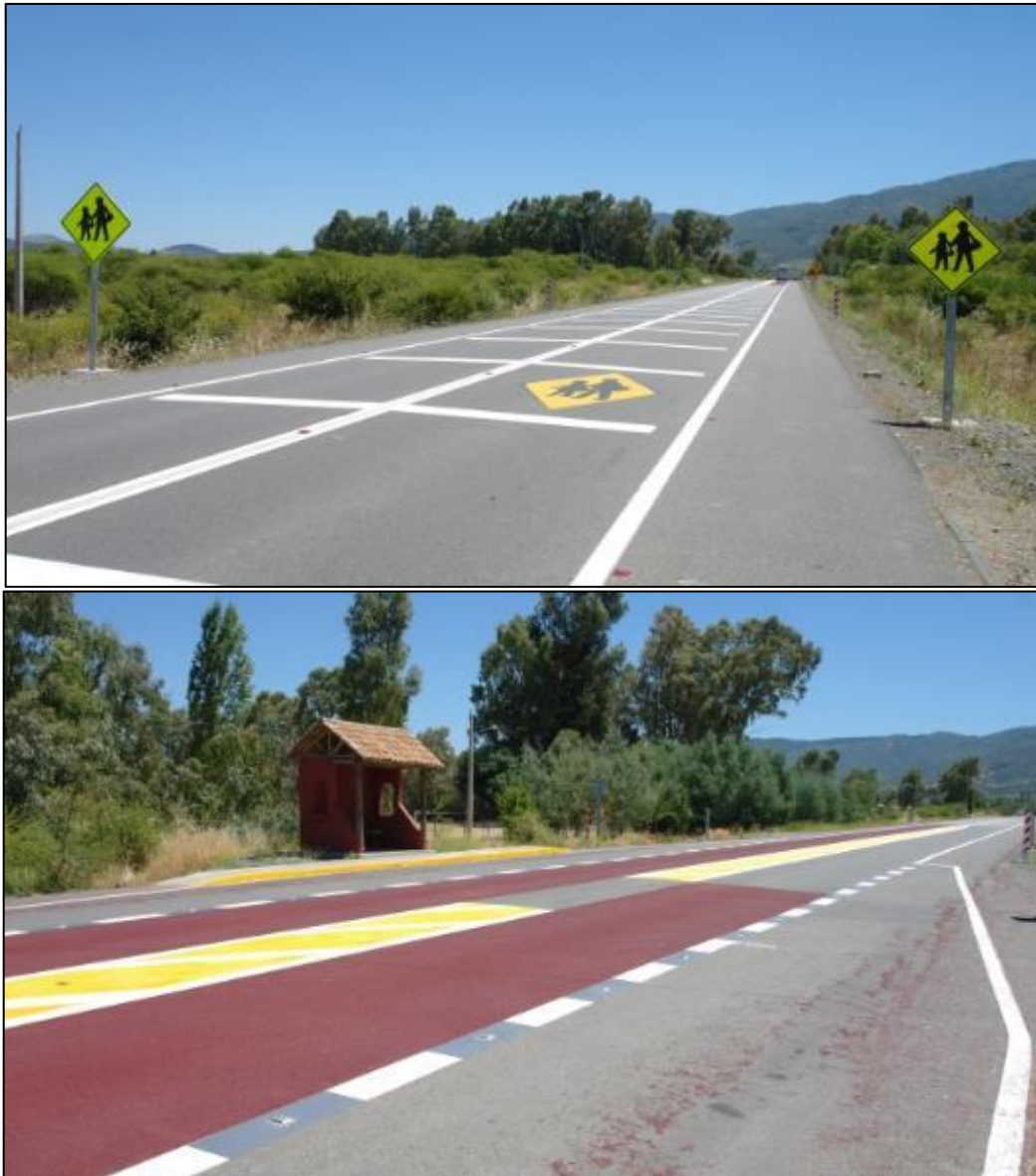
Figure 6.3 - Transverse lines on both lanes and high friction surface, near to (left) and on front (right) the school.
