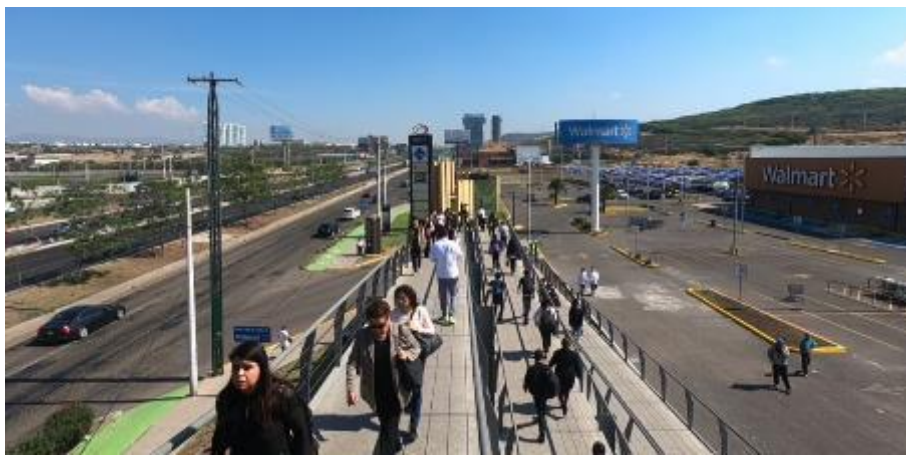
Figure 6.93 - Access ramp to the Pedestrian Crossing-Grade Separation, east side seen from the north view
