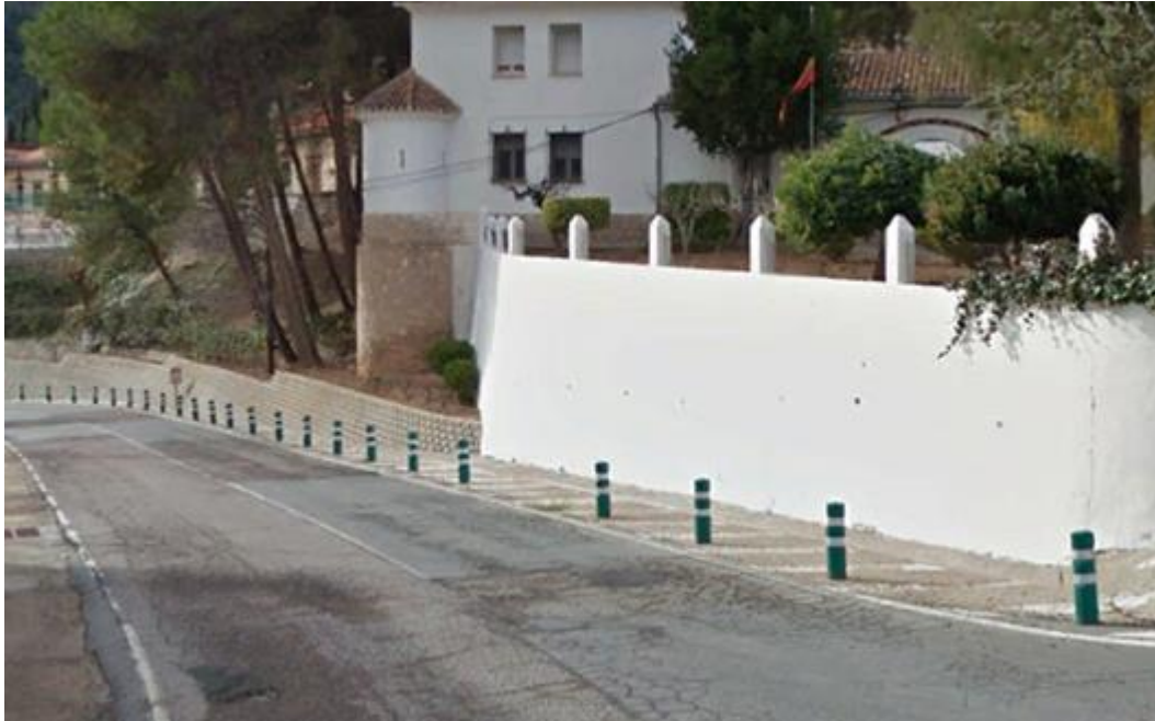
Figure 6.327 - Example of traffic guidance equipment to avoid car parking in zones excluded from traffic
