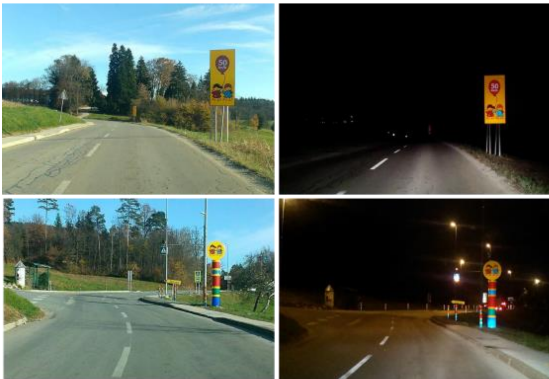
Figure 6.311 - Day / night visibility of information sign, totem and bollards
