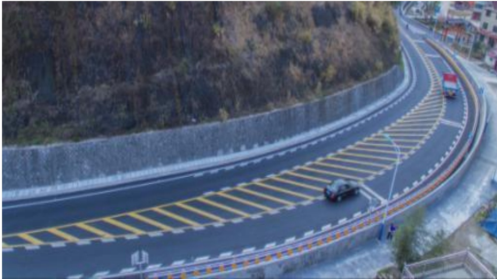
Figure 6.341 - The wider lane and the new virtual canalization island
