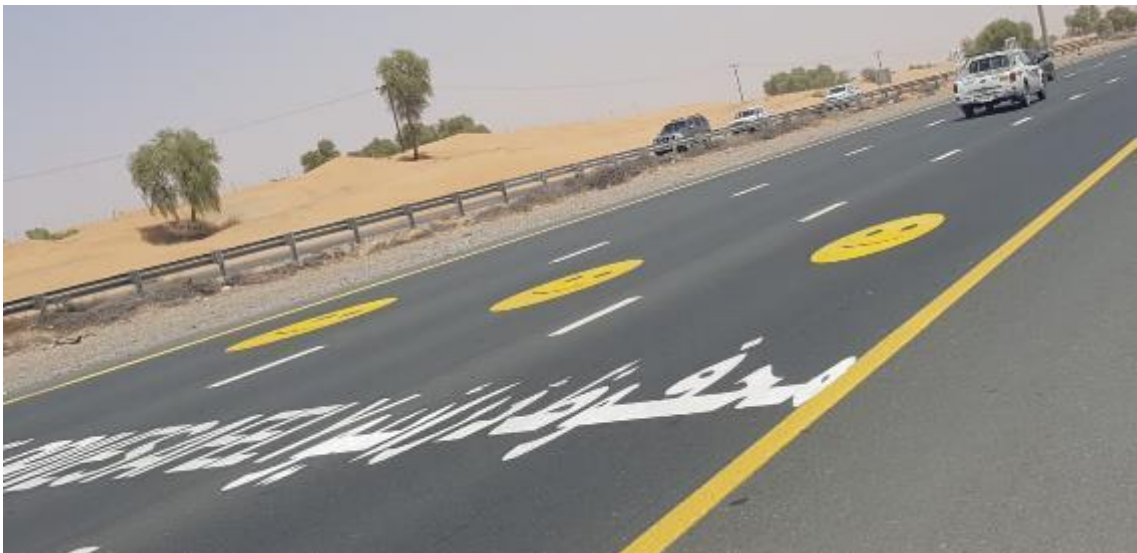
Figure 6.286 - Multilingual motivational road marking for a safe driving. Sheikh Mohammed Bin Zayed Road (Umm Al Quwain). Detail 6
