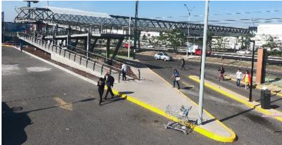
Figure 6.92 - Panoramic view of the permanent Pedestrian Crossing-Grade Separation, seen from the east side
