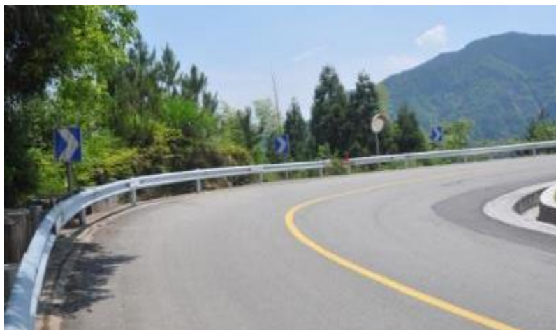
Figure 6.336 - To set guardrails, visual guiding devices, delineators, convex mirrors and other facilities
