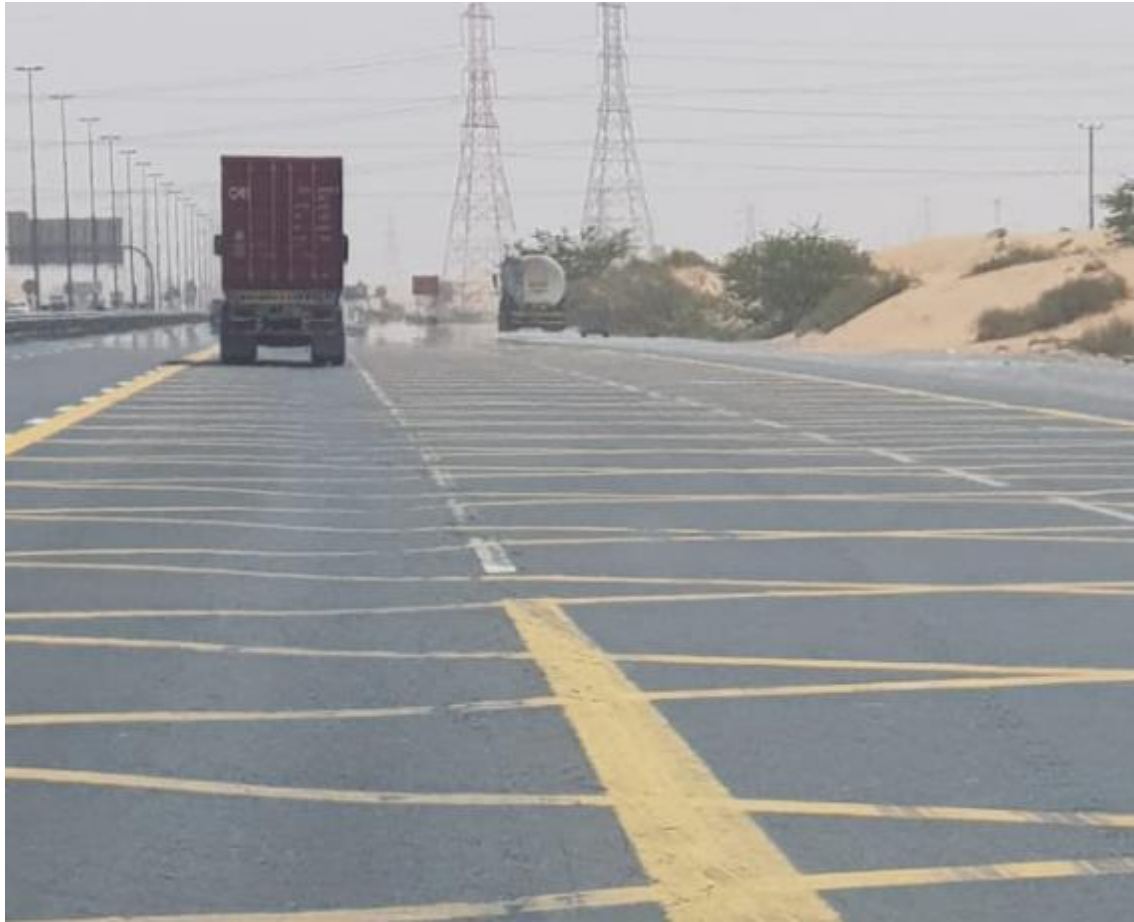
Figure 6.300 - Yellow marks to avoid invasion of heavy vehicles when having traffic jam in the slow lane (increasing of safety from drivers coming from the link road). Detail 5
