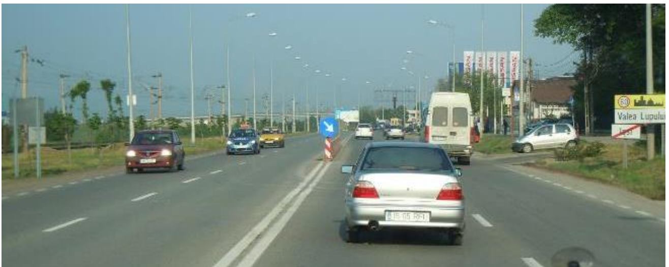
Figure 6.109 – Before the second intervention: road section 2, Valea Lupului oriented view
