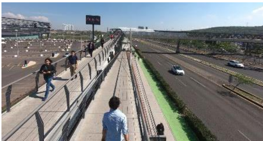
Figure 6.97 - Access ramp to the Pedestrian Crossing-Grade Separation, west side seen from the north view
