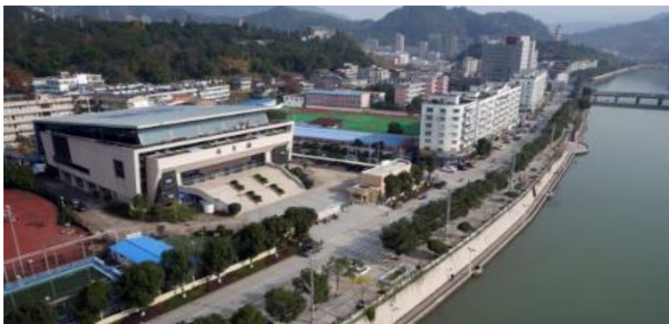
Figure 6.4 - The K56+030 on the G322 line before implementation
