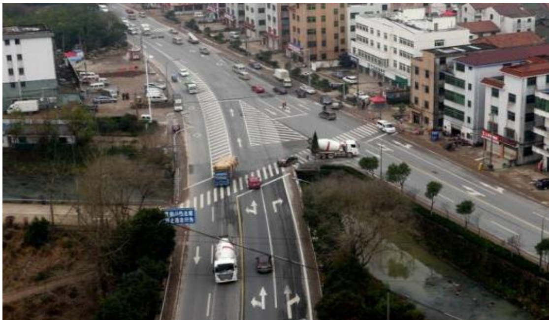
Figure 6.12 - The intersection of S210 and S103 Hangjin line before implementation
