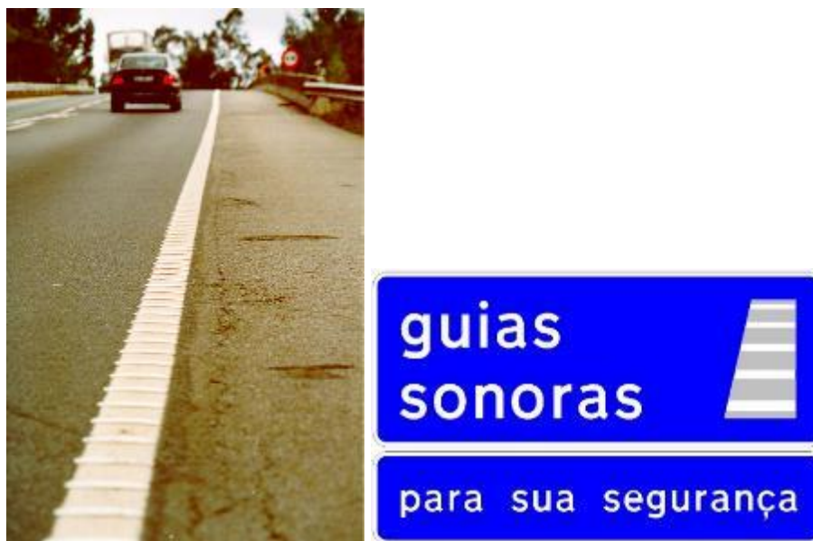
Figure 6.238 - Edge rumble lines and corresponding information sign
