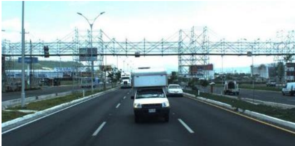
Figure 6.90 - Provisional Pedestrian Crossing-Grade Separation detected during the RSI
