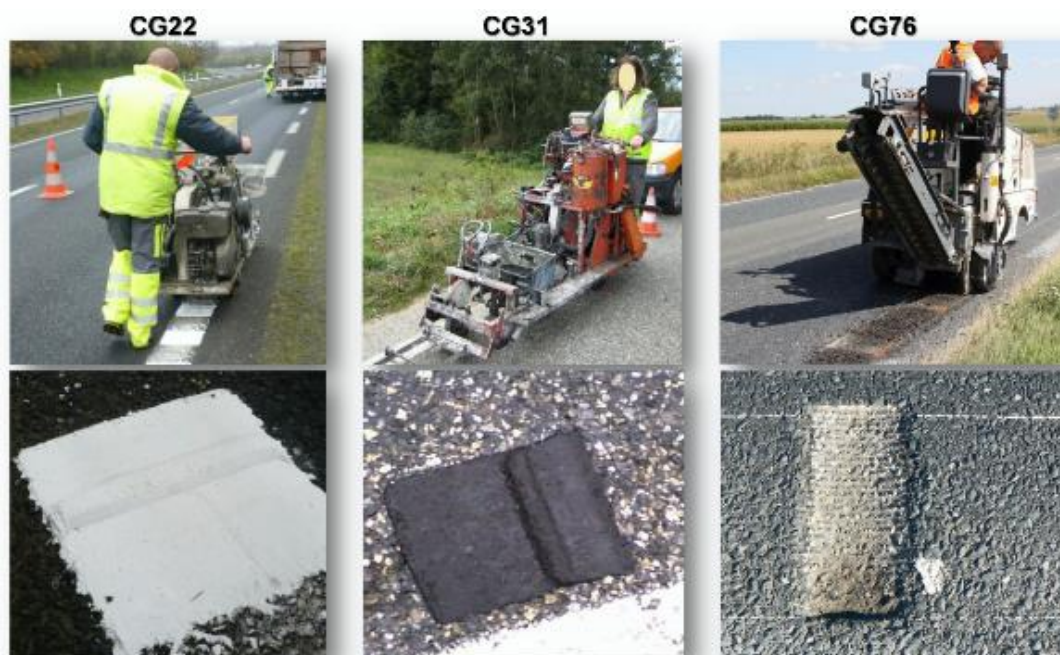
Figure 6.208 - Pictures of implementation of the raised or milled rumble strips for the in situ evaluation. Picture at left: view of the implementation of raised rumble strips for the divided highway in Côte d'Armor (Department 22, France). Pictures at centre: views of the implementation
