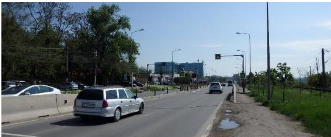
Figure 6.116 – After the intervention: road section 1, Iasi oriented view
