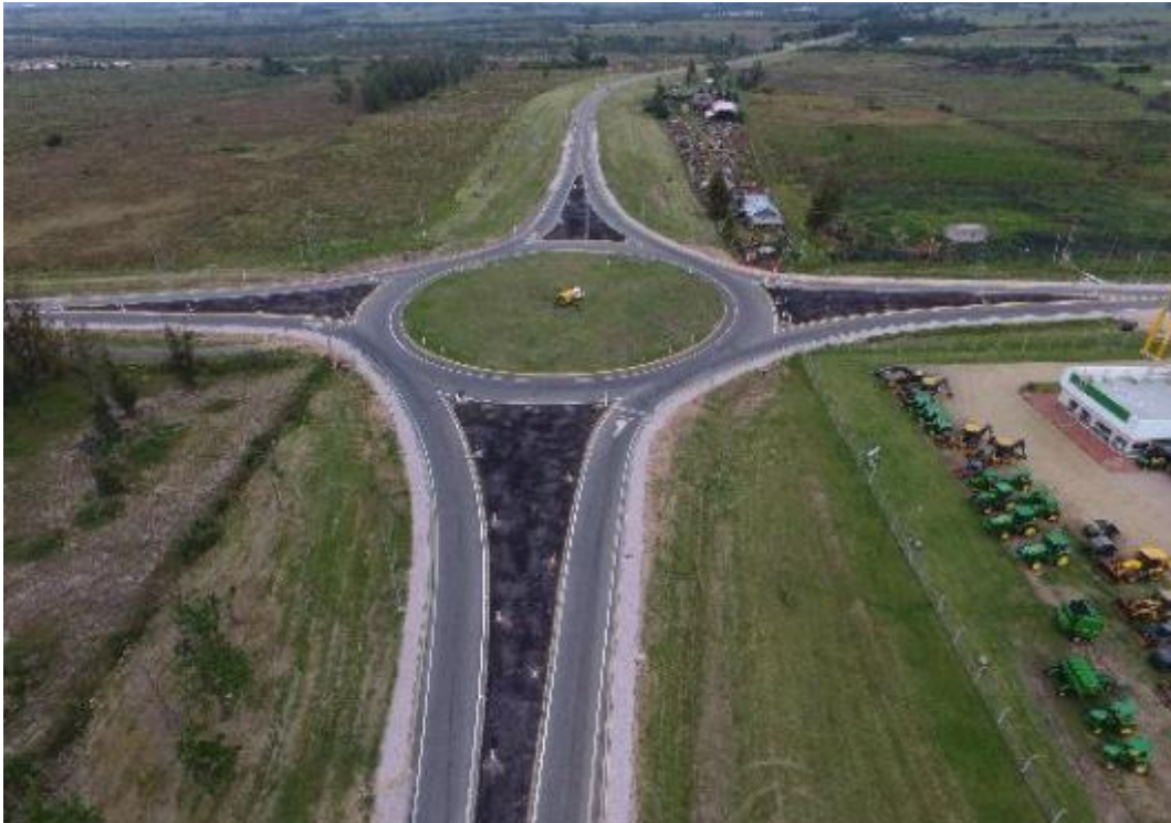
Figure 6.350 - Roundabout Route N° 9 and Route N° 39.
