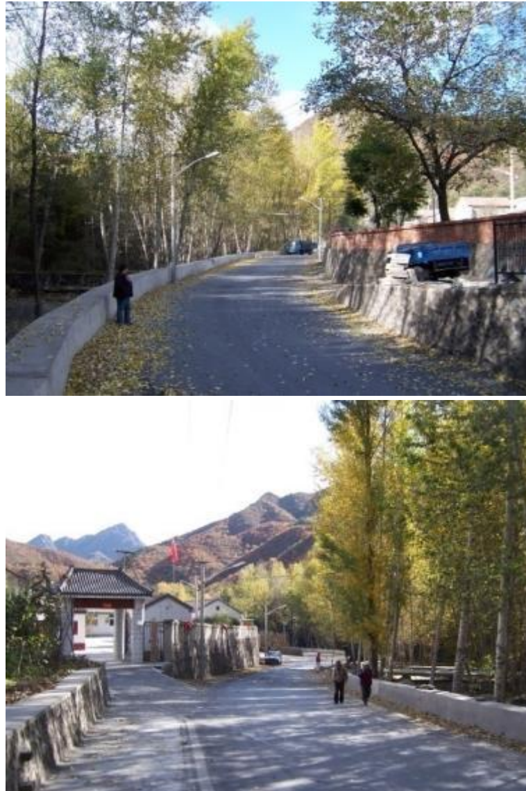
Figure 6.354 - Lack of warning and speed control measures
