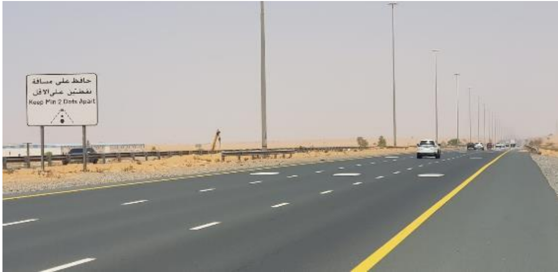
Figure 6.290 - White dots to keep safety distance. Sheikh Mohammed Bin Zayed Road (Umm Al Quwain). Detail 3
