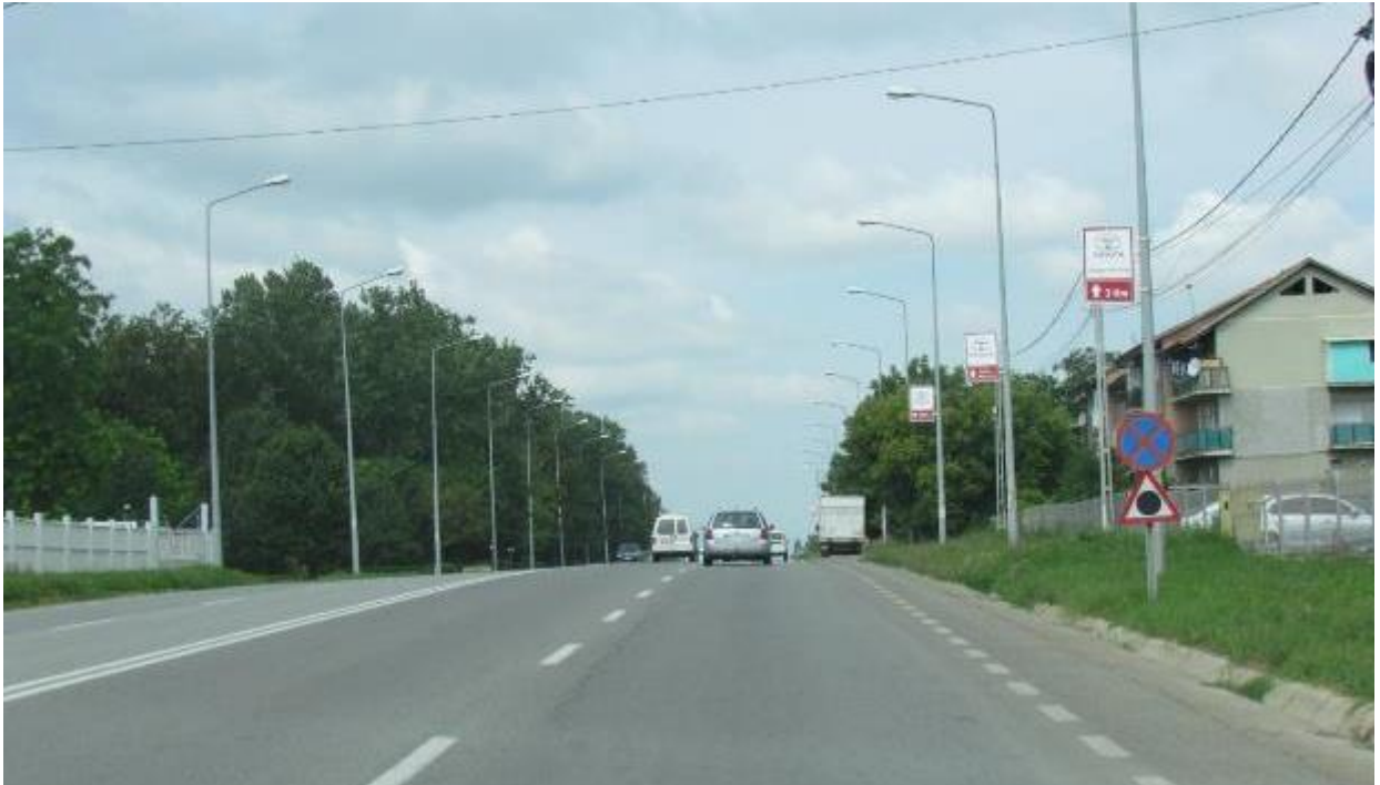
Figure 6.358 – Before the intervention. Road view before the turning point, section 1
