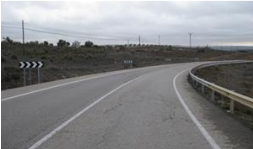
Figure 6.280 - Example of site clearing to improve sight in curve
