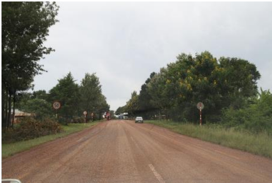
Figure 5.4 - Linear settlement with no physical 'gateway' or change in cross section though village
