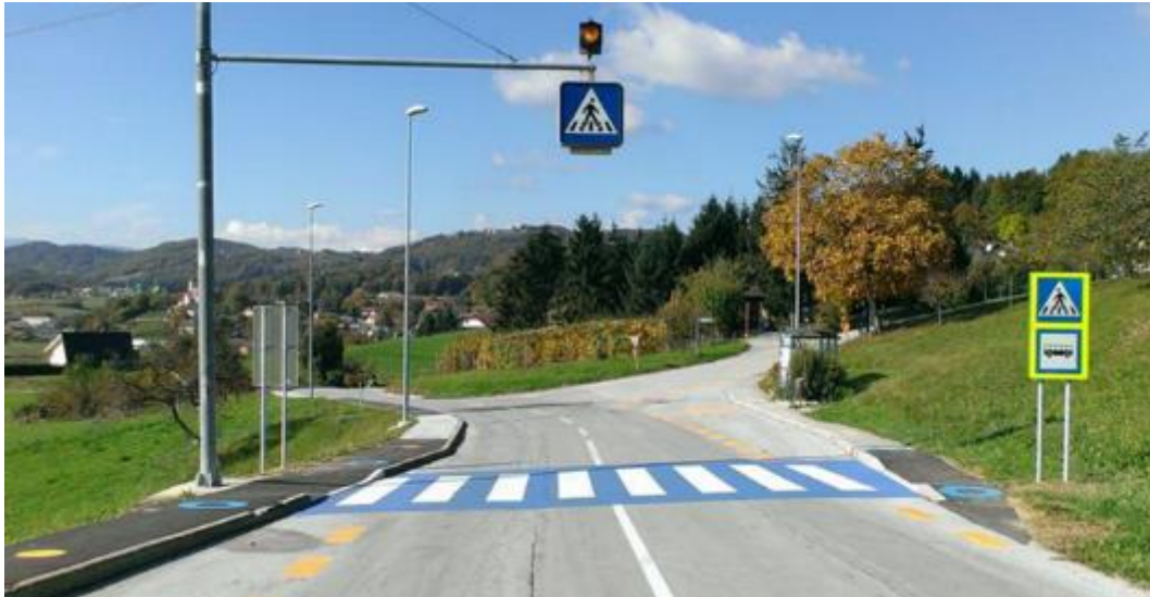
Figure 6.310: Pedestrian crossing on blue contrast and new traffic sign
