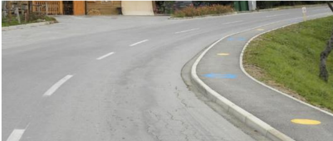
Figure 6.307: Pavement markings (blue and yellow circles)
