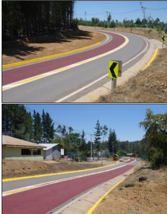
Figure 6.1 - Lane narrowing on horizontal curve with high friction surface, near to (left) and on front (right) the school.
