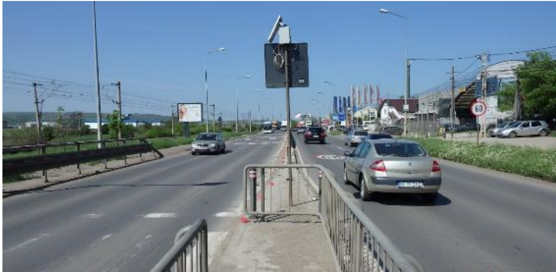
Figure 6.115 – After the intervention: road section 1, V Lupului oriented view, details of the pedestrian refuge island
