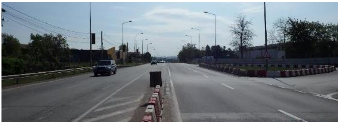
Figure 6.363 – Turning point after the intervention
