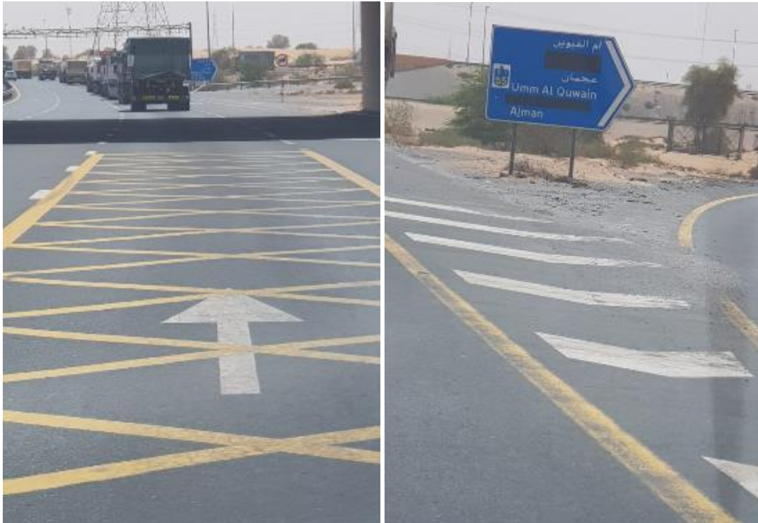
Figure 6.297 - Yellow marks to avoid invasion of heavy vehicles when having traffic jam in the slow lane (increasing of safety from drivers coming from the link road). Detail 2
