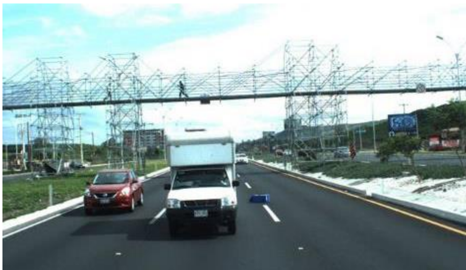
Figure 6.91 - Detail of pedestrians using the provisional Pedestrian Crossing-Grade Separation
