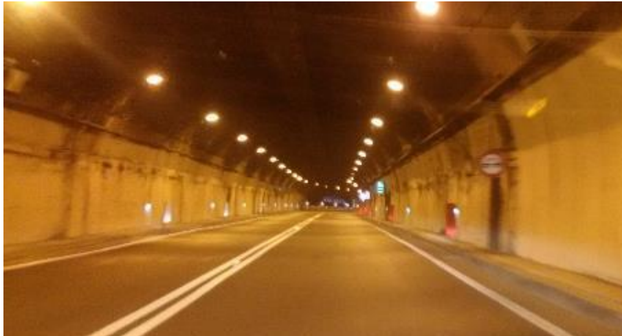
Figure 6.214 - Tunnel internal view with visual obstacles at the entrance and interection of the secondary road
