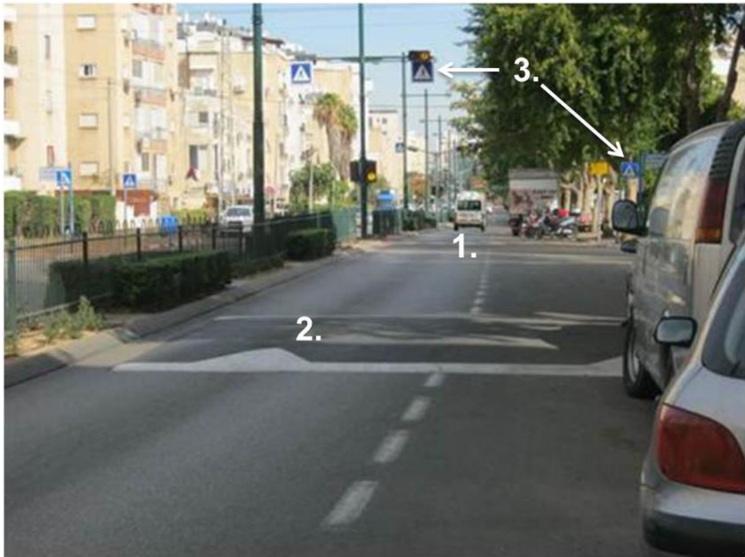
Figure 6.59 - Main components of a raised crossing arrangement, on the example of Site B in Israeli study.
