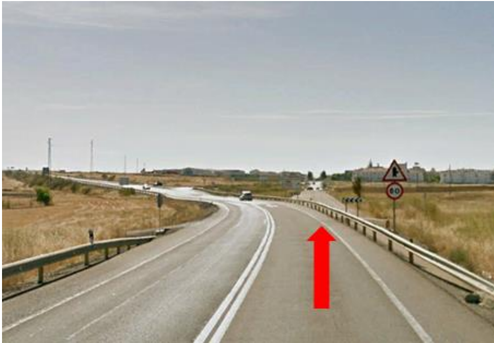
Figure 6.271 - N-432 ordinary road. West junction of Llerena. Secondary road is in extension of the main road
