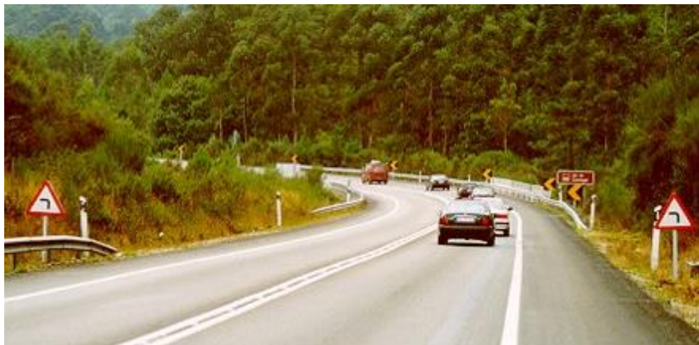
Figure 6.237 - Curve signing with danger warning and chevron alignment signs
