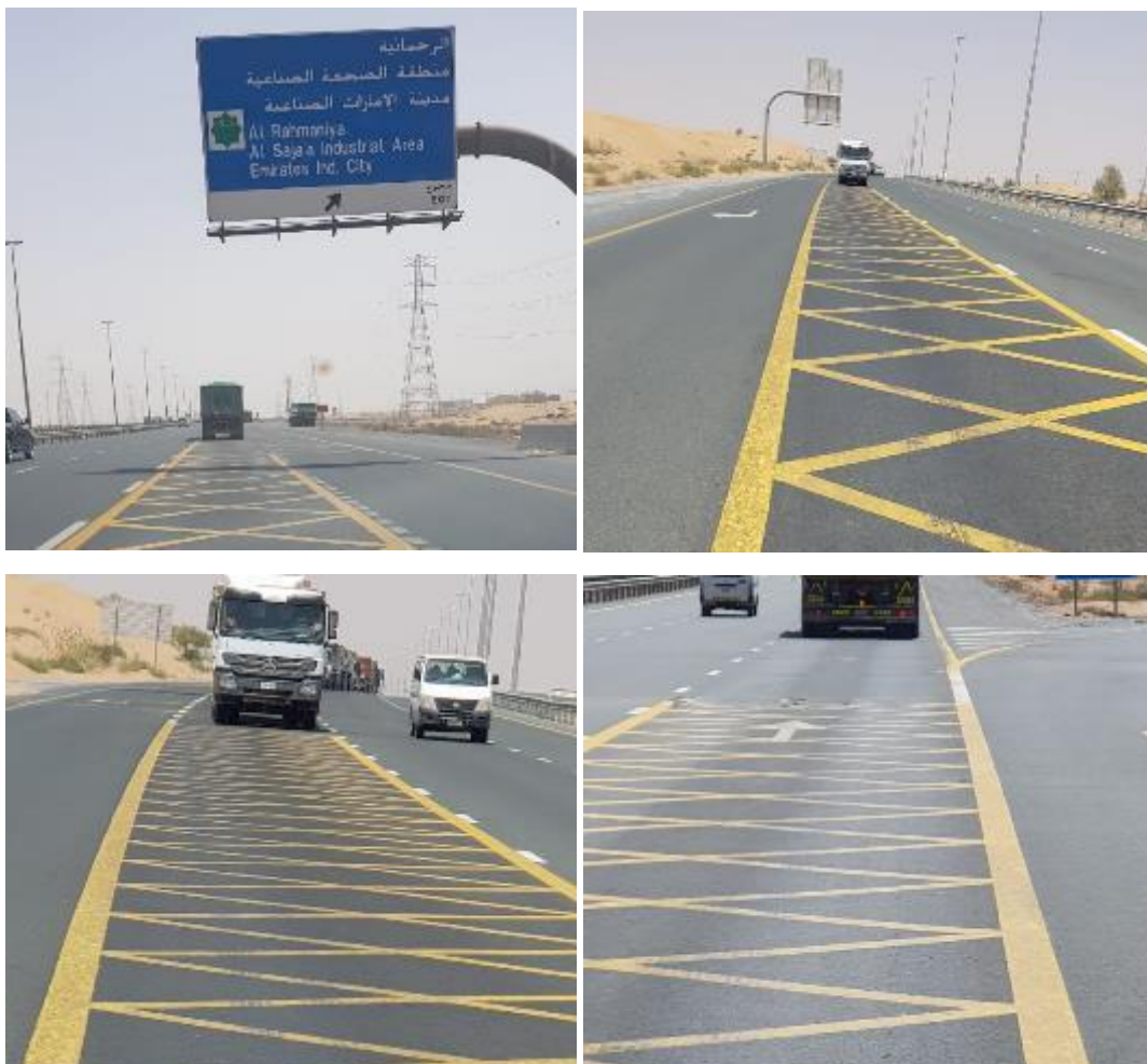
Figure 6.296 - Yellow marks to avoid invasion of heavy vehicles when having traffic jam in the slow lane (increasing of safety from drivers coming from the link road). Detail 1
