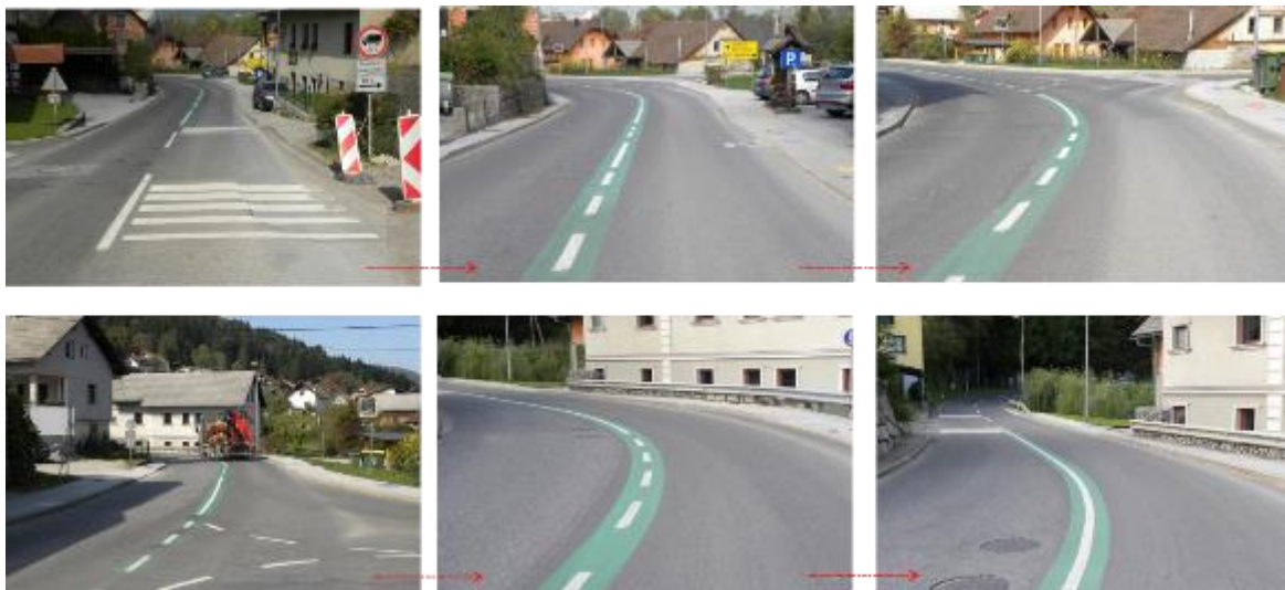
Figure 6.262 – Site after the intervention, Direction B
