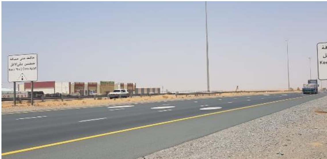
Figure 6.288 - White dots to keep safety distance. Sheikh Mohammed Bin Zayed Road (Umm Al Quwain). Detail 1
