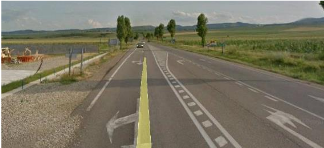
Figure 6.179 – View from the road after the intervention, closer to the intersection 2
