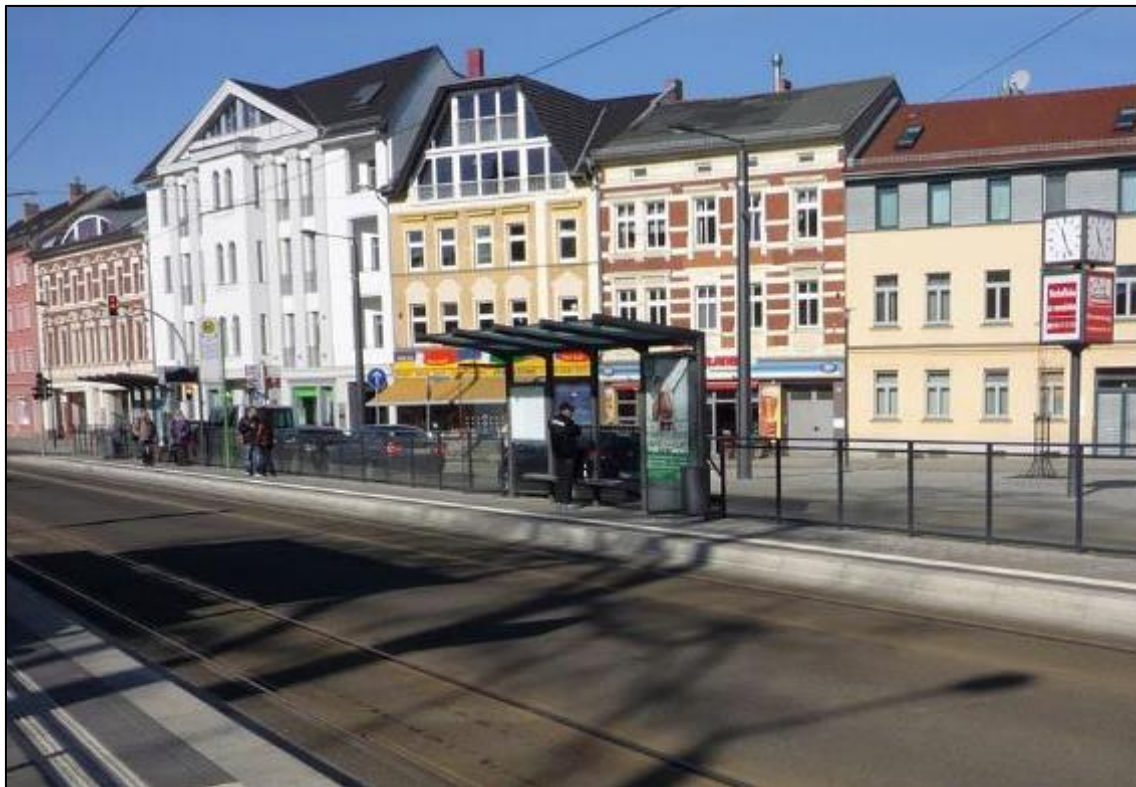
Figure 6.20 - New combined tram/bus stop in the western arm of the junction (Source: www.teamteibrant.de )
