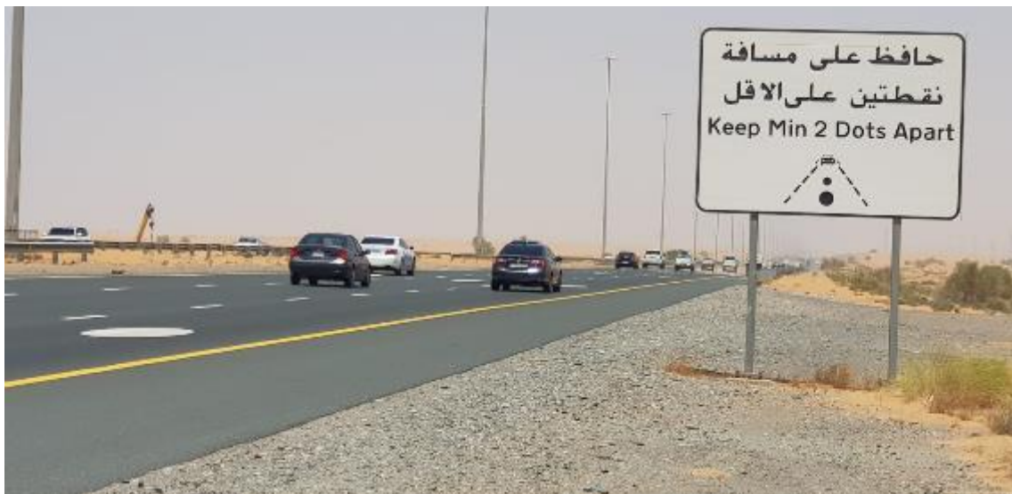
Figure 6.293 - White dots to keep safety distance. Sheikh Mohammed Bin Zayed Road (Umm Al Quwain). Detail 6
