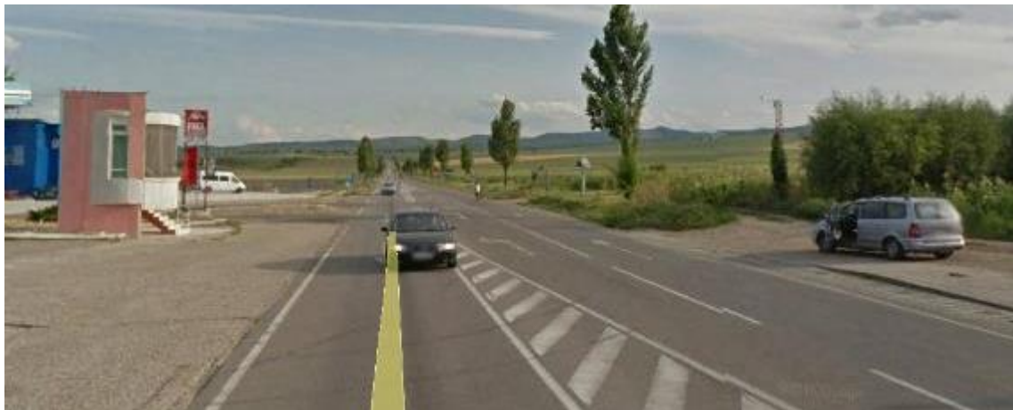
Figure 6.177 – View from the road after the intervention
