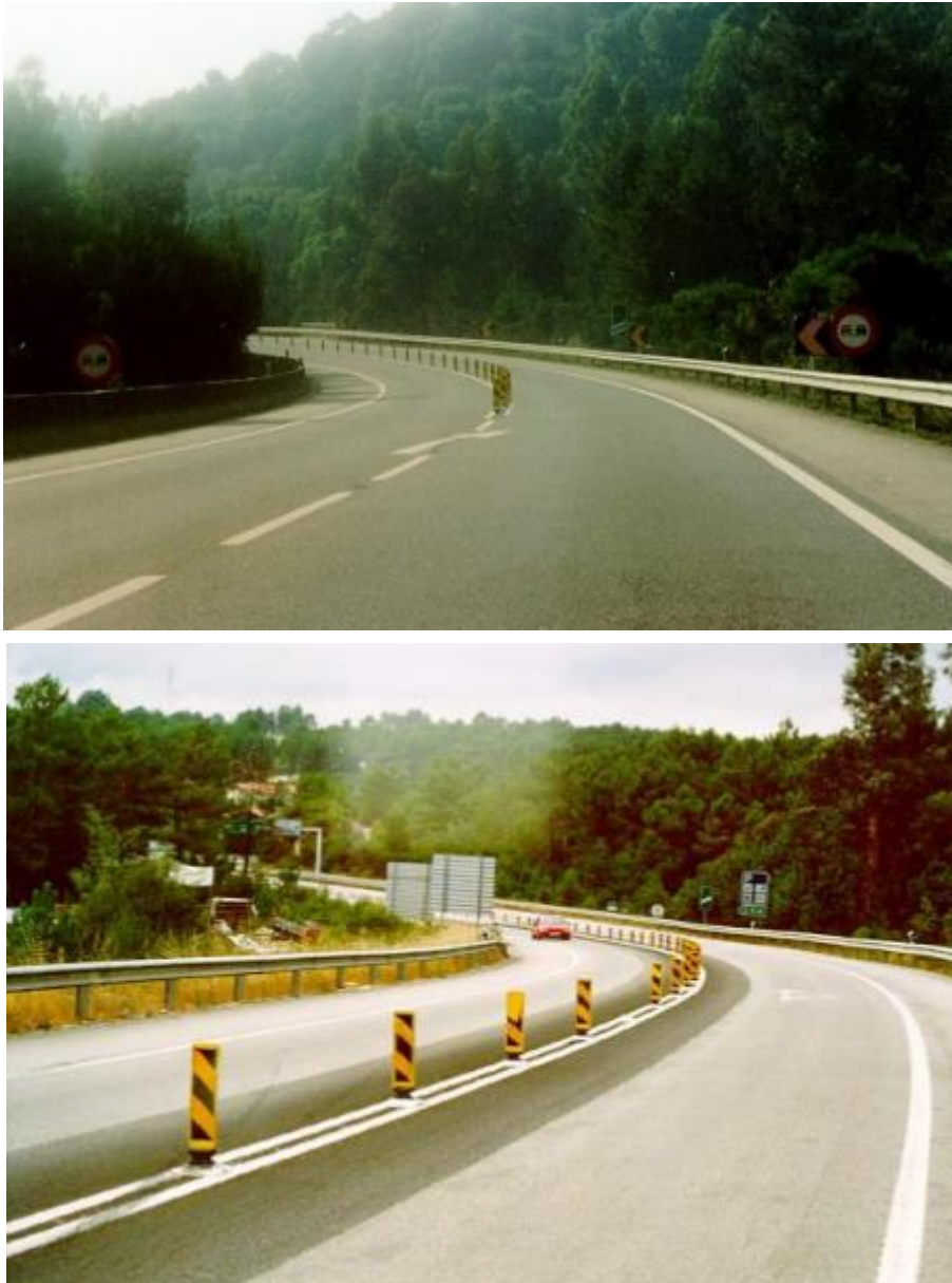
Figure 6.166 – Visual extension of the median to the beginning of the curve in two interchanges
