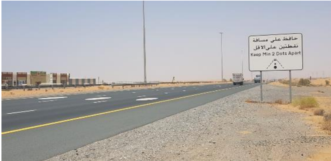
Figure 6.292 - White dots to keep safety distance. Sheikh Mohammed Bin Zayed Road (Umm Al Quwain). Detail 5
