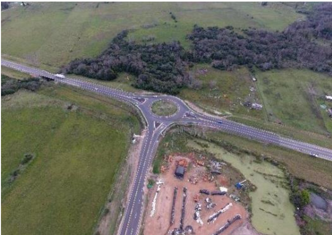
Figure 6.351 - Roundabout Route N° 9 and Route N° 104.
