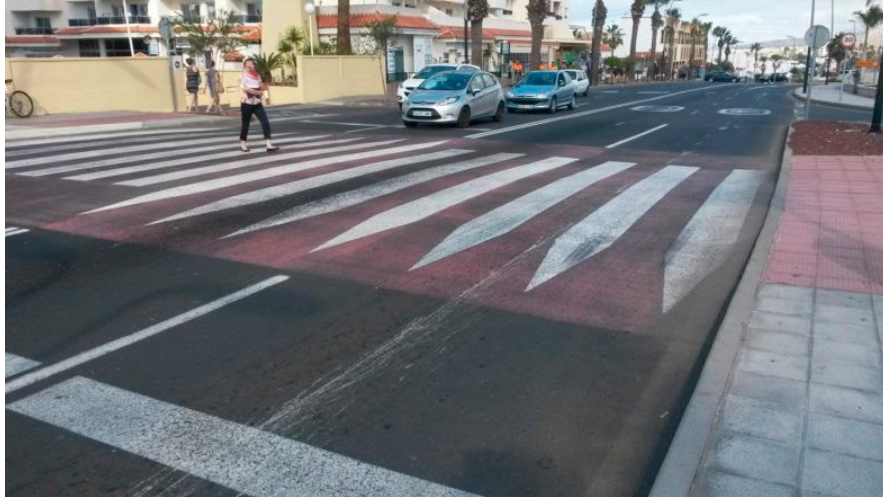
Figure 6.60 - Speed-reducing devices and stop lines or yield bars 8 to 10 m before the crosswalk Playa de las Americas Arquitecto Gomez Cuesto, Tenerife.
