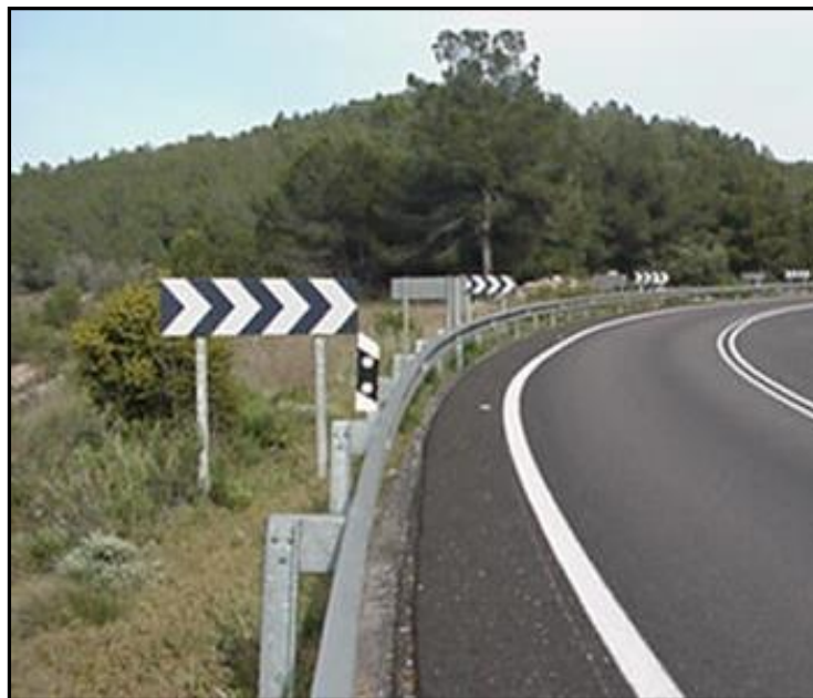
Figure 6.332 – Example of implemented road chevrons
