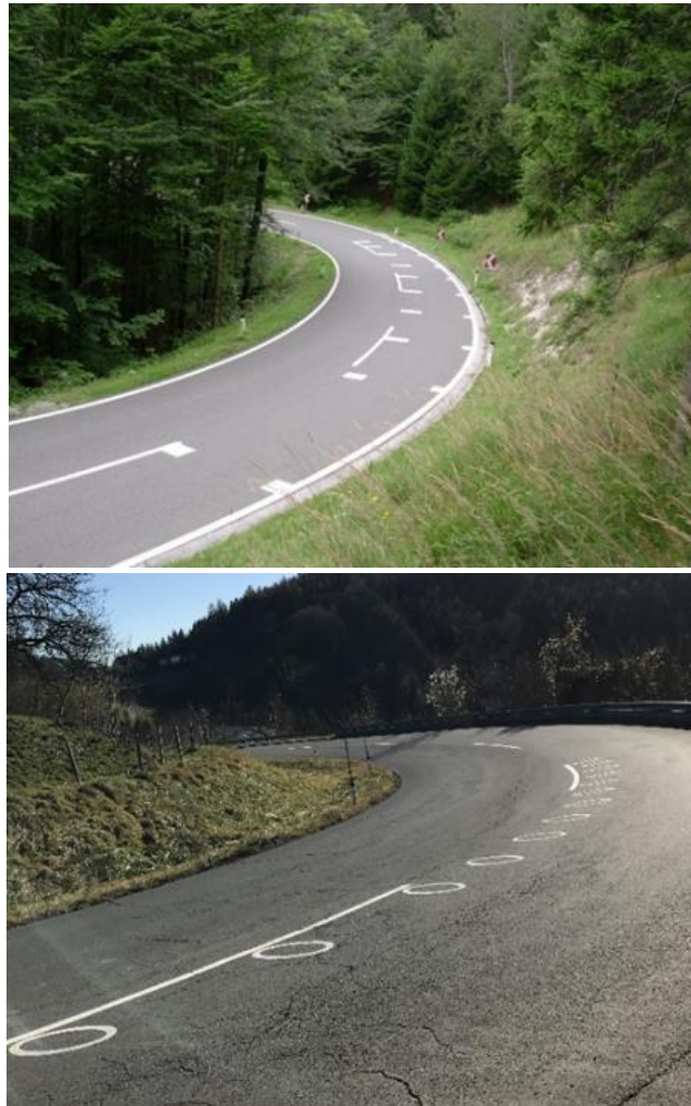
Figure 6.182 - a) “bar” (or “psychological brake”) layout, b) elliptic design
