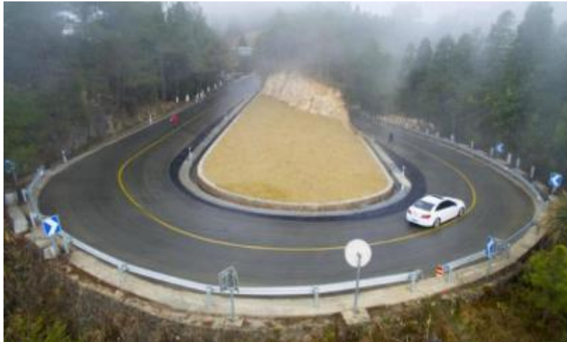
Figure 6.337 - The full view of the road after completion
