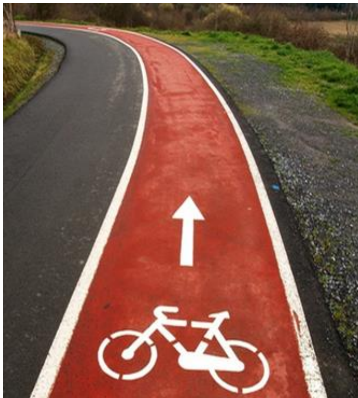
Figure 6.151 - Example of differentiated coloured pavement and specific road marking in a bicycle path
