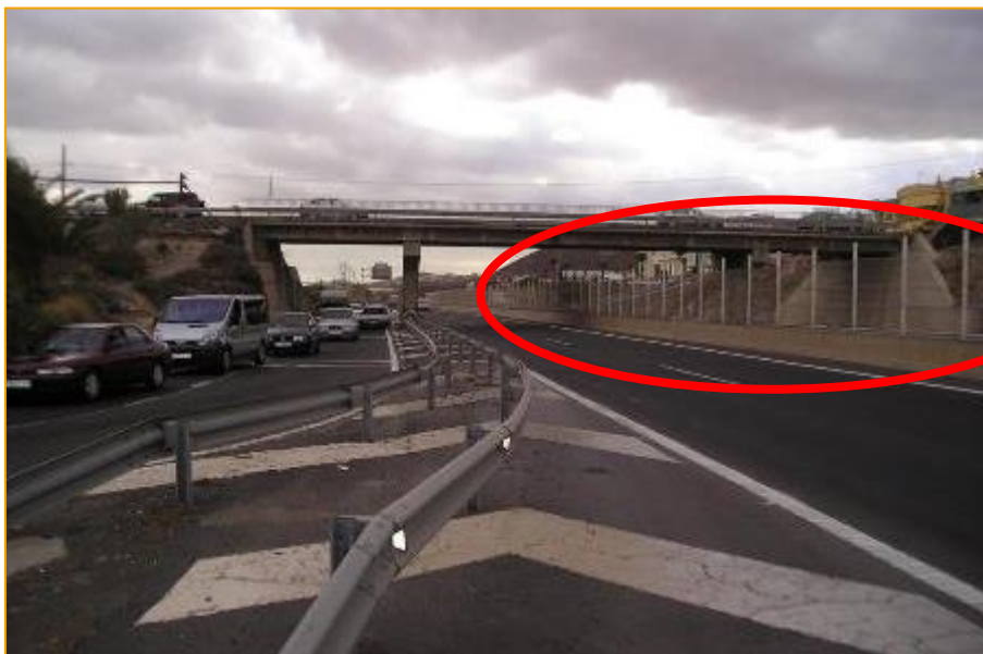
Figure 6.144 - Example of fence over New Jersey barrier, to avoid pedestrian crossing in an area with overpass
