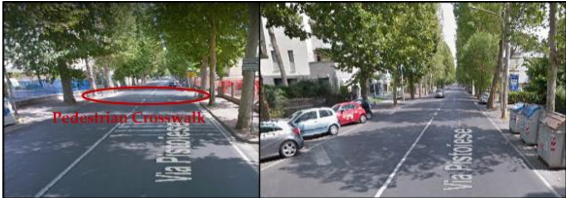
Figure 6.157 - Details of the road before the interventions: on the left, crosswalk with low visibility; on the right, the evidence of wide lanes and long straight. In both cases the trees contribute to move the focal point to the horizon [6].
