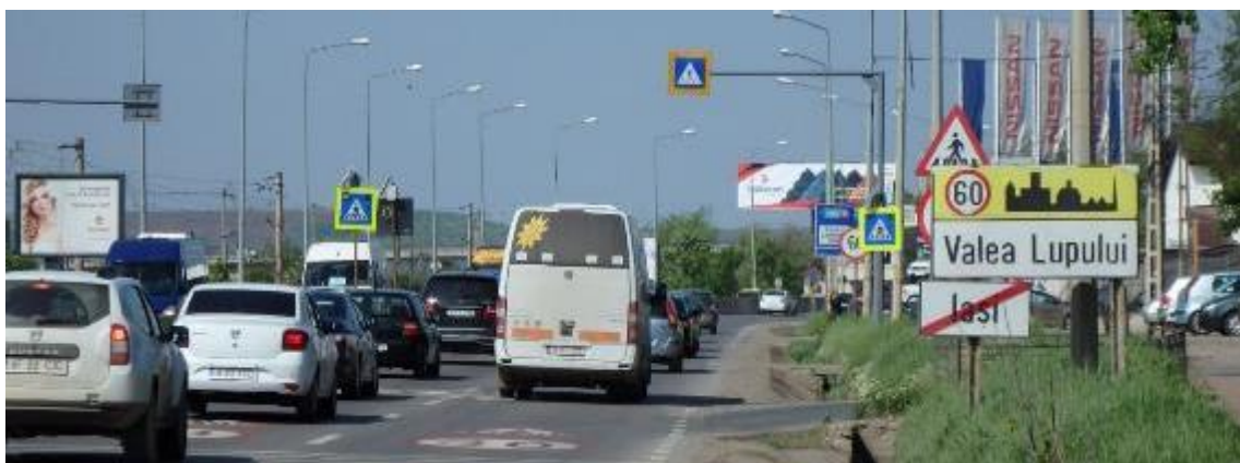
Figure 6.113 – After the intervention: road section 2, V Lupului oriented view
