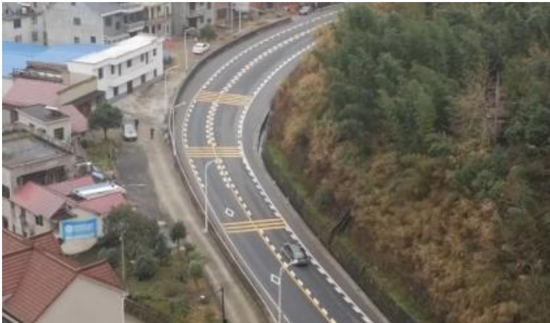
Figure 6.340 - A full view of the road section before the implementation
