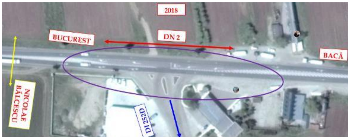
Figure 6.173 – Detailed view of the site after the intervention
