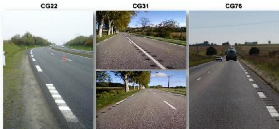
Figure 6.209 - Pictures of implemented raised or milled rumble strips for the in situ evaluation. Picture at left: view of the implemented raised rumble strips on the bend for the divided highway on the dotted road marking of shoulder, in Côte d'Armor (Department 22, France). Pictures at centre: views of the implemented raised rumble strips of colour pavement, at upper, raised rumble strips were implemented from either side of centreline marking on the dotted road marking. At lower, they were along the left side of shoulder markings in Haute-Garonne (Department 31, France). Picture at right: views of the milled rumble strips were shoulder rumble stripEs (i.e., marking is placed over the rumble strips) in Seine-Maritime (Department, 76, France).
