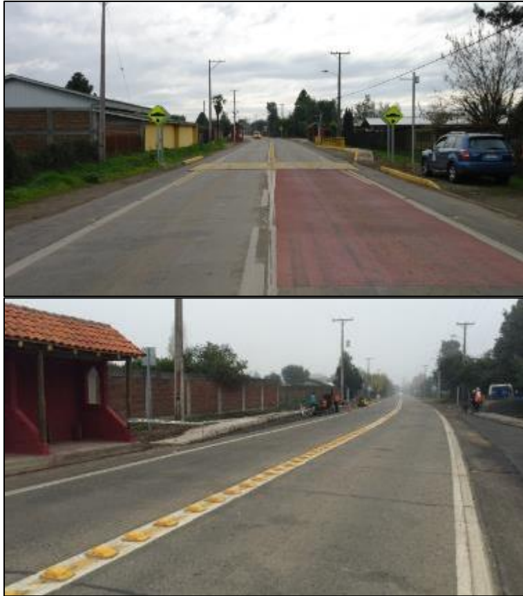
Figure 6.2- Speed hump (5 cm height), near to (left) and on front (right) the school.
