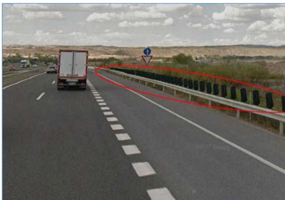
Figure 6.276 - Anti-glare screen on metal safety barrier
