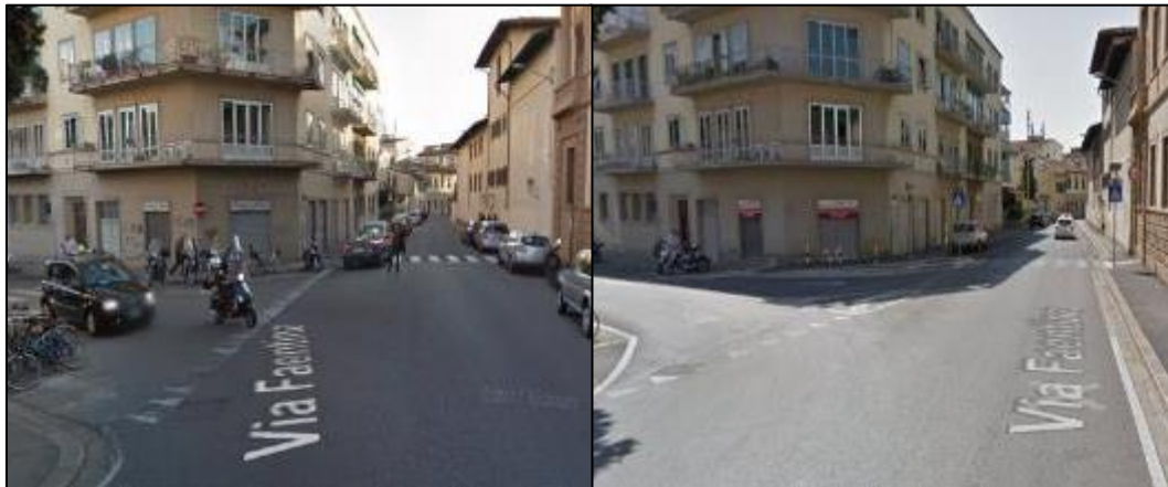
Figure 6.87 - Site 3, on the left situation before the intervention, on the right situation after the intervention [2]
