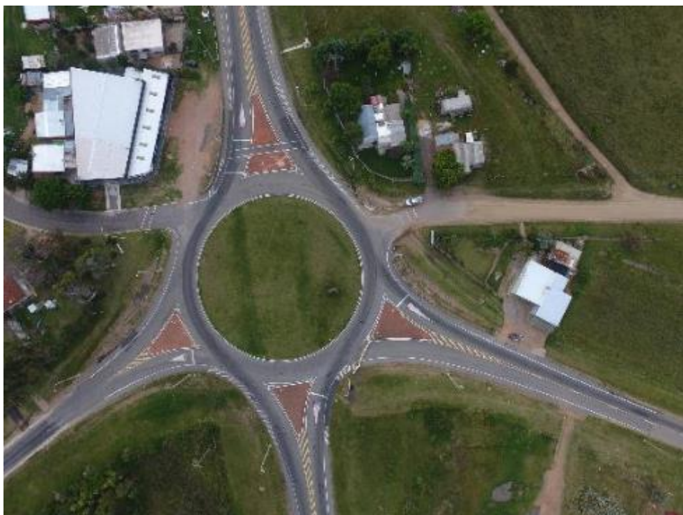
Figure 6.349 - Roundabout Route N° 9 and Route N° 37.
