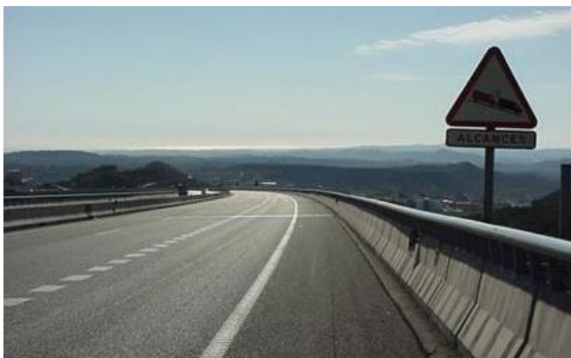
Figure 6.319 - A-3 high way, kilometer point 316 (Valencia). P-31 vertical sign with complementary board
