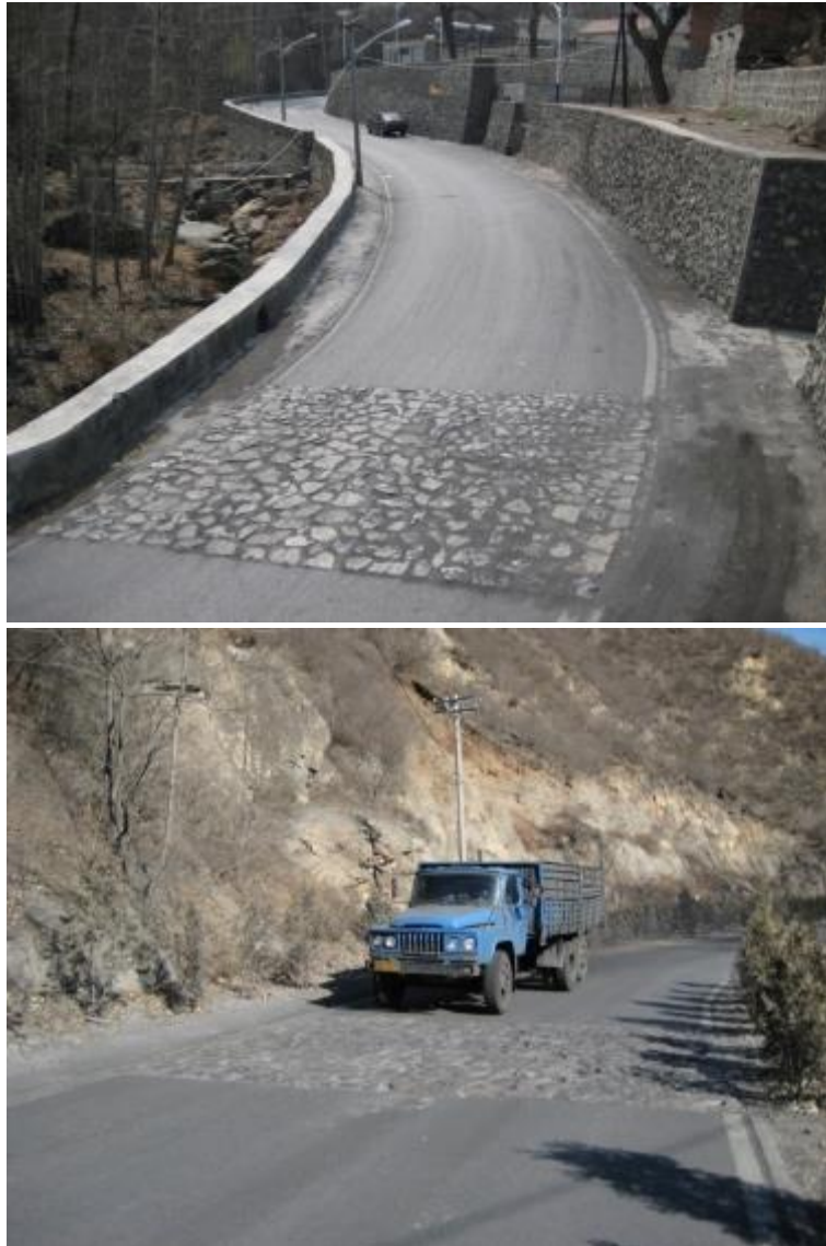
Figure 6.355 - The dimension stone pavement section in the front of the entrance to Xidamo village
