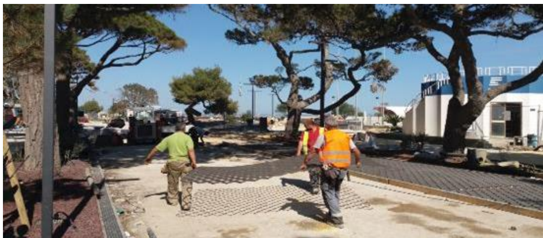
Figure 6.225 – Reconstruction of road paving
