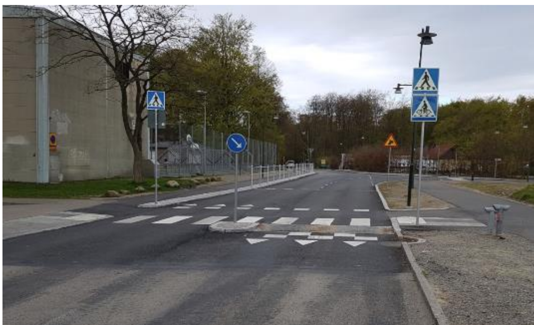
Figure 6.135 - Realization of a bicycle crossing with pedestrians crossing and speed reduction (speed humps). Source: City of Helsingborg
