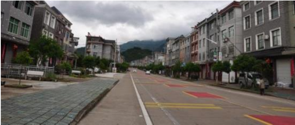
Figure 6.8 - Lay the coloured antiskid pavement and deceleration vibration markings
