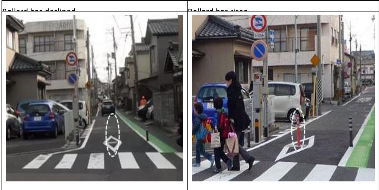
Always descending except in the traffic regulation time zone. Large vehicles (excluding micro) can not be passed at all times Figure 6.89 - Installation status of Soft Rising Bollard. Made by MLIT HP Regulations on traffic on weekdays 7: 30-8: 15 (school time zone) http://www.mlit.go.jp/road/road/traffic/sesaku/torikumi.html#2-2-4
