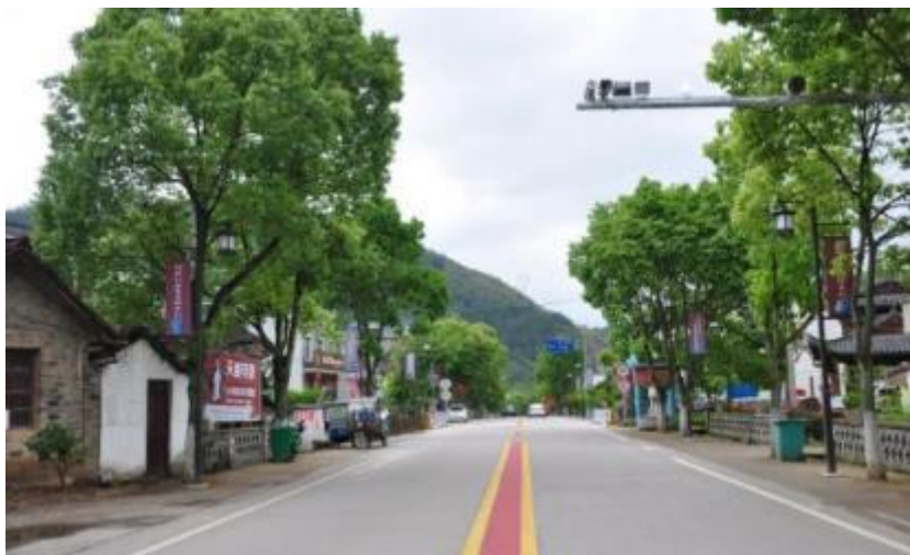
Figure 6.201 - the camera and road monitoring system
