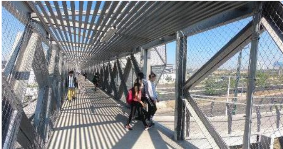
Figure 6.95 - Interior view of the Pedestrian Crossing-Grade Separation
