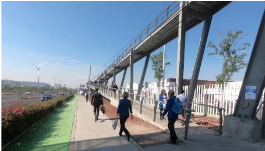
Figure 6.96 - Access ramp to the Pedestrian Crossing-Grade Separation, west side seen from the south view
