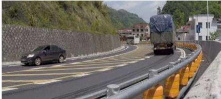
Figure 6.343 - The crash barrier after the implementation
