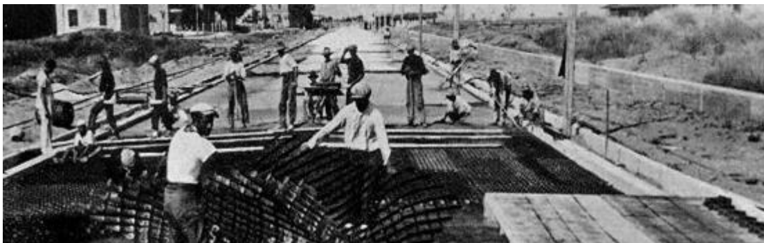
Figure 6.224 – Construction of original road paving
