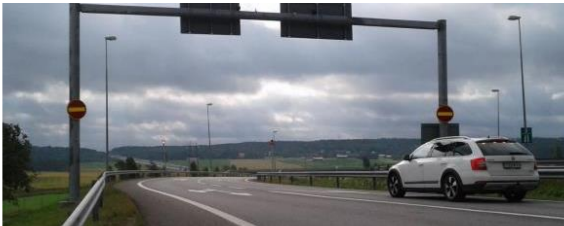
Figure 6.207 - The most significant system developed in the new project were warning lights that turns red if a driver is about to take a motorway ramp in the wrong direction. Photo: Jaakko Klang
