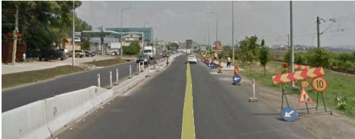
Figure 6.112 – During the intervention: construction site section 1, Iasi oriented view
